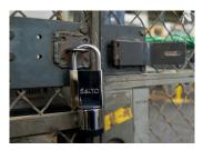
A GEO Padlock was installed on the front gate of the courtyard. The GEO Padlock sounds exactly what it is - a card reader on a padlock. This means that employees with the right authorization can still access the courtyard at predetermined times while maintaining the security of the facility. Hager also uses this on the sliding door gate into the Intertek testing facility. The area must be kept secure to comply with testing regulations.
