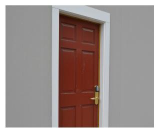
Four exterior doors required updating, and the wide body escutcheon was chosen. These four doors did require some alteration for the new locking mechanism; however, it only required two 9/16" holes drilled in each door.
